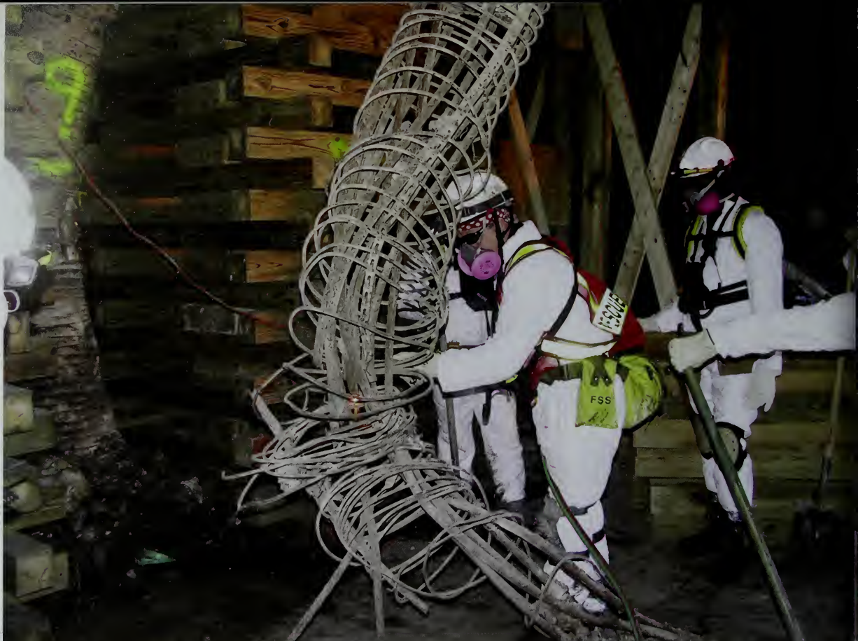
Above: Removing a damaged building column.
